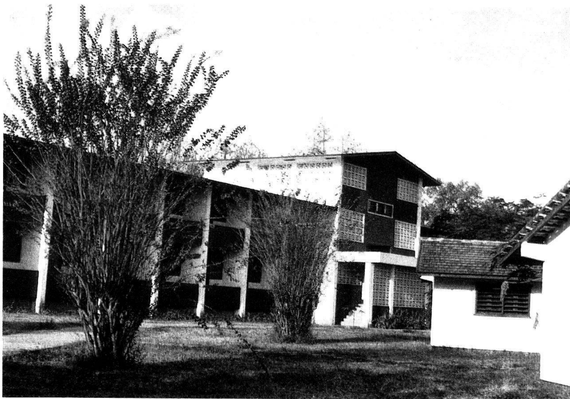
Fig. 3. South façade of the students hostel at Ifakara.
