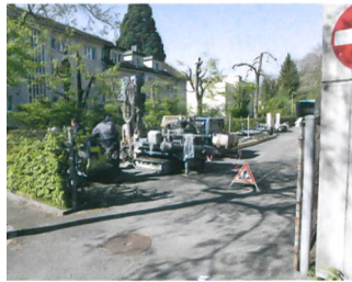
75 Nidau, AGGLOlac/Neue Station, Mühleruns
