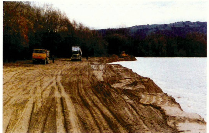
Shore before and during rubble filling.
