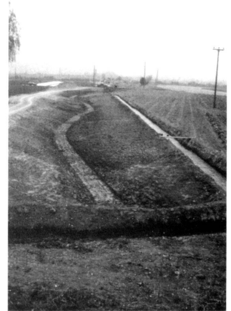
Left: When this stream was shifted and reconstructed, compact sections of the narrow, high-growing herbaceous borders were removed in packages and kept in store for further use (approx. 6 months).
