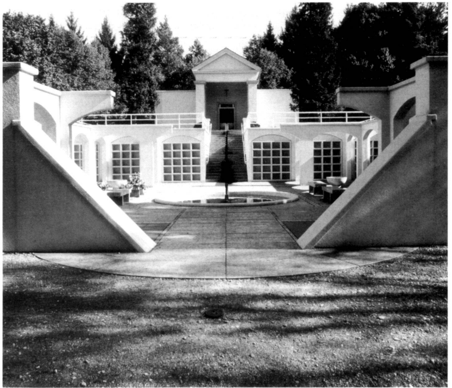
Urnenanlage Waldfriedhof Singen. Fotos: P. Horn, Stuttgart Colombarium du cimetière forestier de Singen. Urn burial area, Singen forest cemetery.
