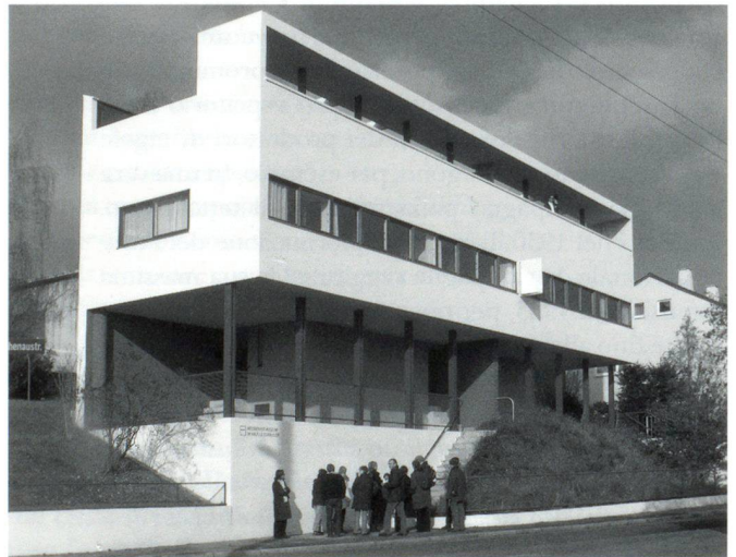
Weissenhofsiedlung, Stoccarda, Le Corbusier House, 1927.
