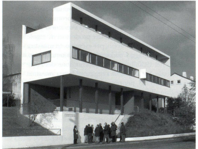
Weissenhofsiedlung, Stoccarda, Le Corbusier House, 1927.
