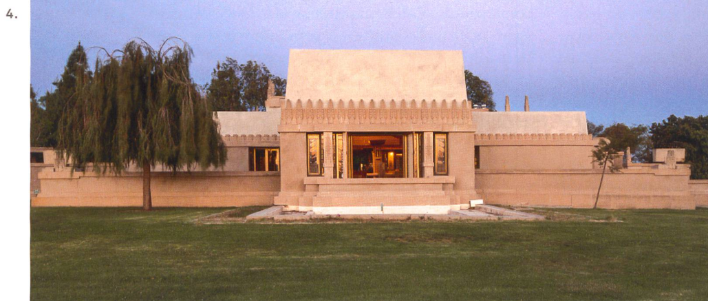
3. Hollyhock House, pianta. Fonte K. Smith, Frank Lloyd Wright. Hollyhock House and Olive Hill , Rizzoli, New York 1992, p. 80 4. Hollyhock House, esterno. Foto Joshua White / JWPictures.com
