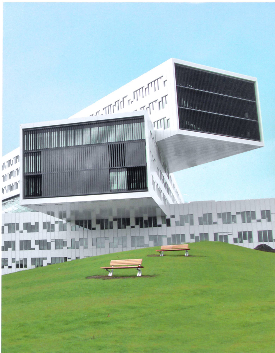
Statoil Headquarters, Oslo
