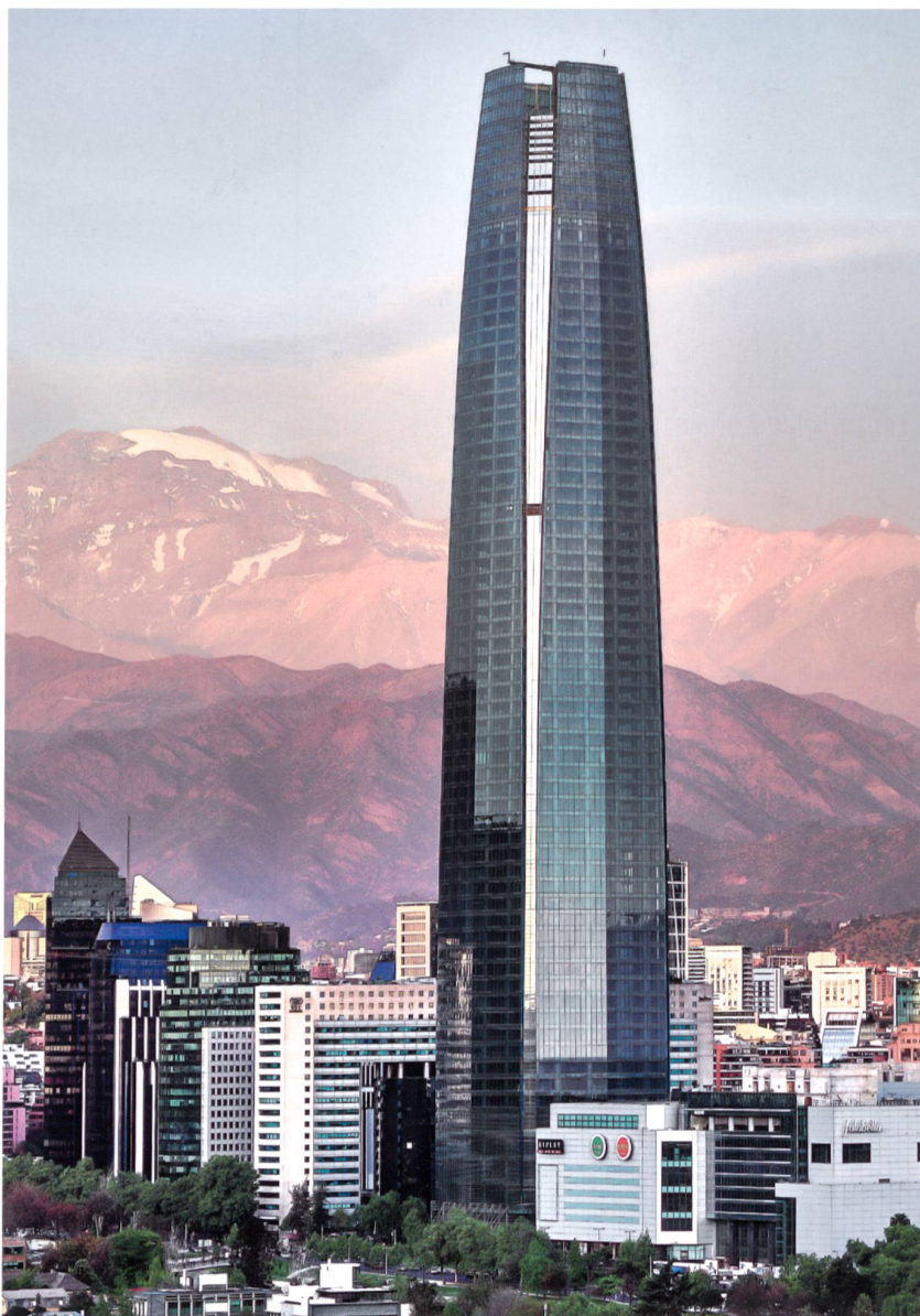
Costanera Center, Santiago, Chile
