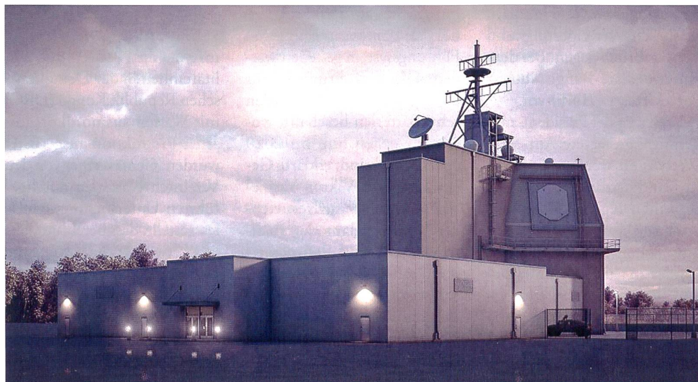
AEGIS ASHORE-System in Deveselu.
