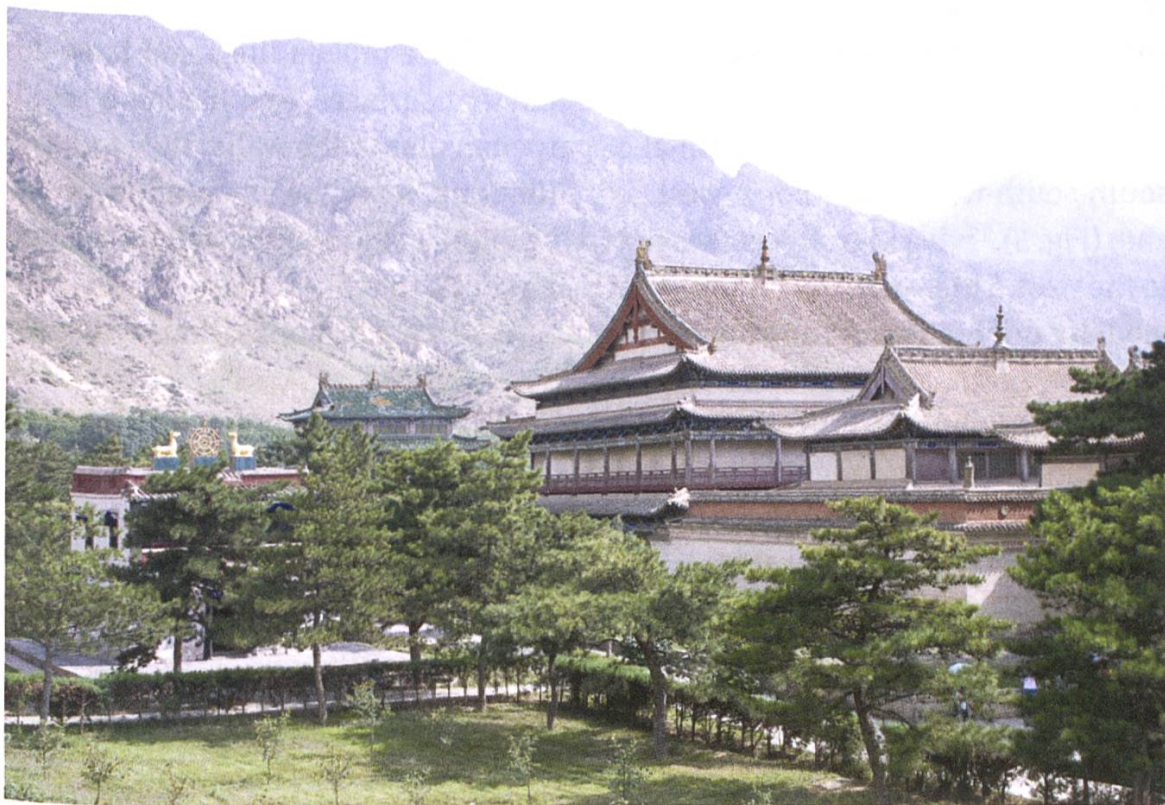
Fig. 4: Main Assembly Hall and Liulidian in the background and on the left, the small Tibetan-style Nayicung Temple
