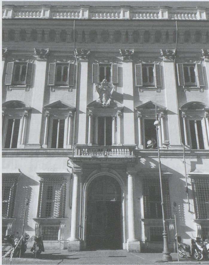
Fig. 11: Palazzo Chigi, Rome, 1664–1667, detail of central bays and entrance (photo: author).
