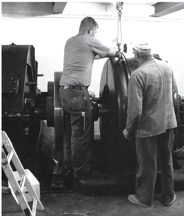
Renovation des Generators.
