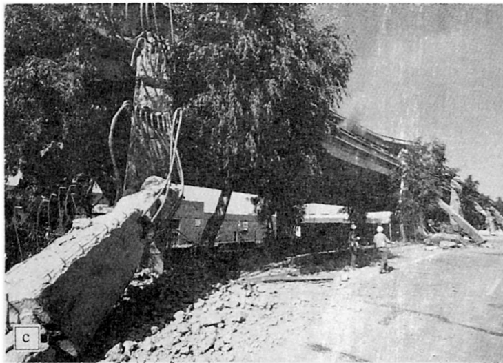
FIG 1. Bridge Damage During the 1989 Loma Prieta Earthquake
