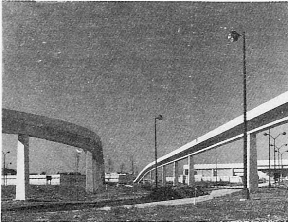
Fig 6. Straight stems and curved decks offer economy during construction at the Dallas/Fort Worth Airport.
