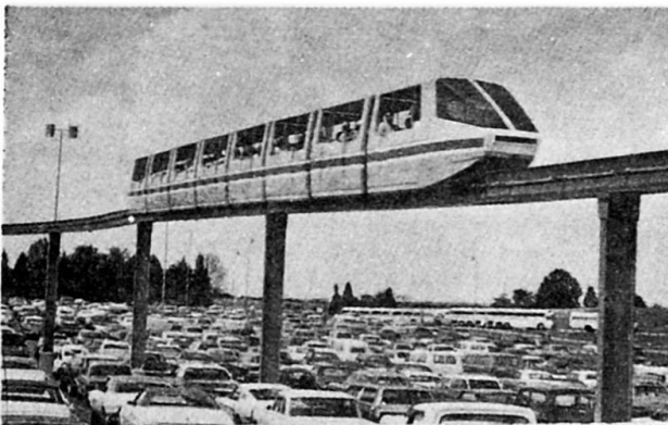
Fig. 2 Westinghouse Guideway Kings Dominion, Virginia
