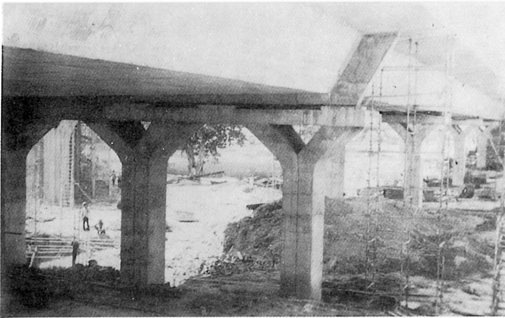
Fig. 5 Flyover Portion 'ABCD'
