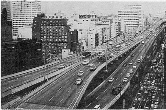
Fig. 4 Semba Rooftop Expressway: Osaka
