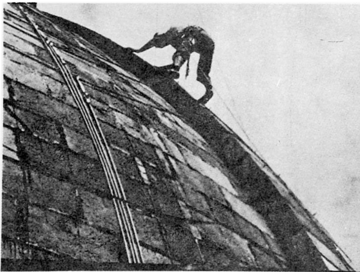
Pic.33: The operations to place the cables
