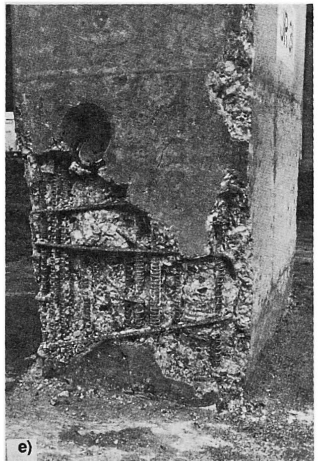
Fig 3. Bridge Damage, Loma Prieta 1989 (M7.1)
