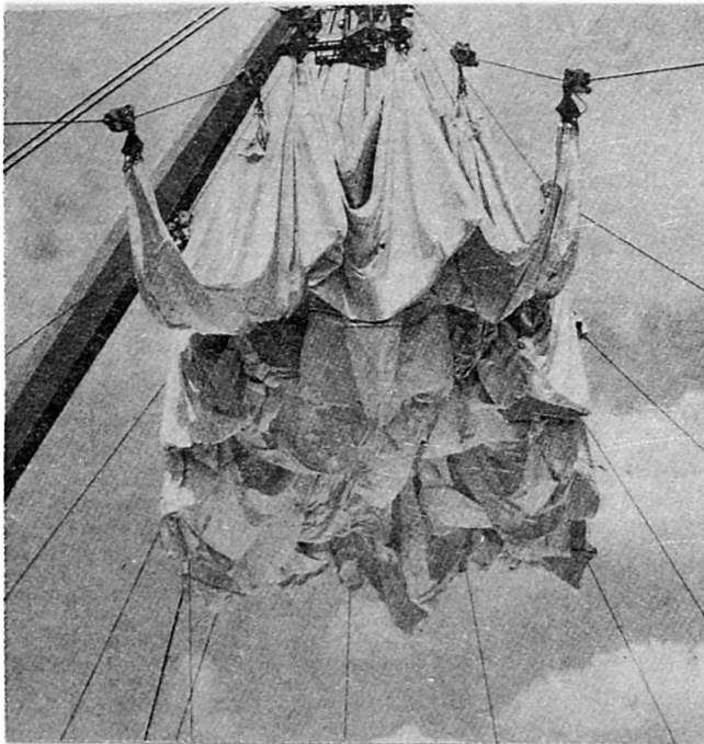
Fig. 2 Swimming Arena Düsseldorf Membrane roof in open-air posi- tion; the tractors have pulled up the membrane edges along the main cables.
