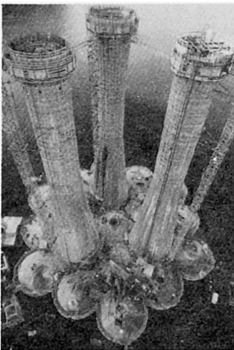
Fig. 5 Platform TCP2 under construction in Norwegian Shipyard
