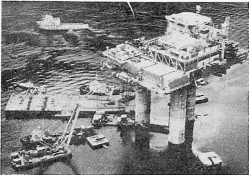
Fig. 3 Platform TCP2, during construction
