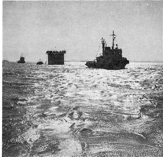
Fig.2 Caissons being towed in sea
