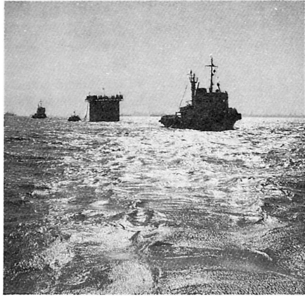
Fig.2 Caissons being towed in sea
