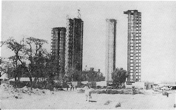
Fig.10 Slipformed Lift Cores
