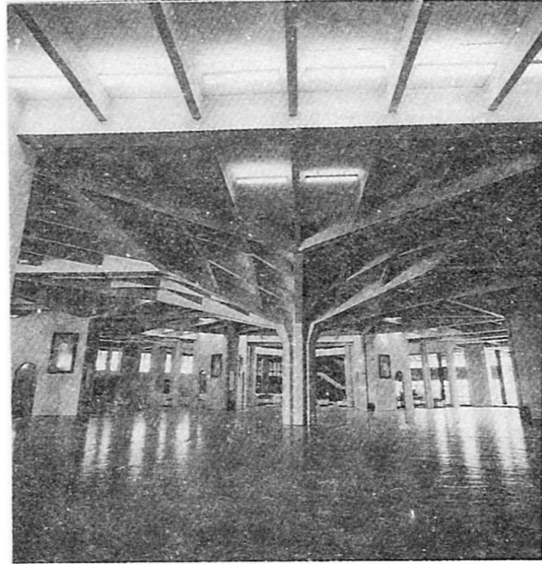
Fig.6 The stylised flower supporting Assembly Floor
