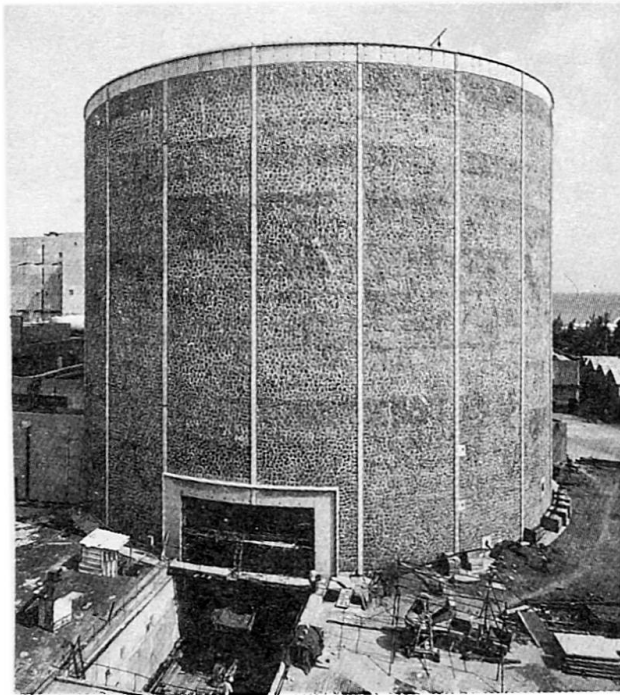
Fig.6 View of completed reactor, Madras
