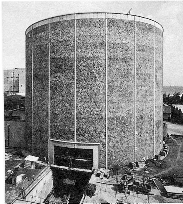
Fig.6 View of completed reactor, Madras
