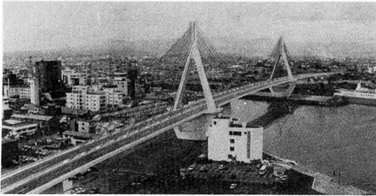
Fig. 5 Photomontage of completed Aomori Bay Bridge
