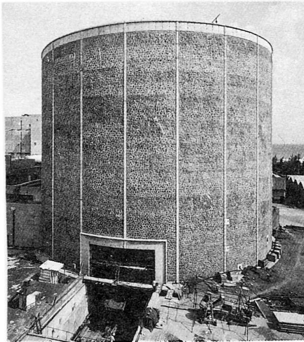
Fig.6 View of completed reactor, Madras
