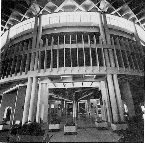
Fig.24 Assembly hall, Gandhinagar
