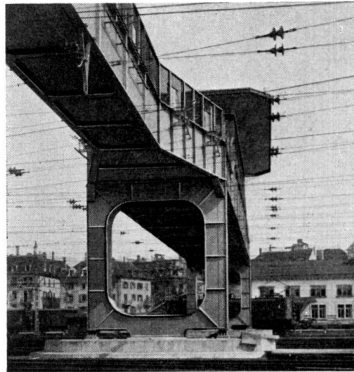
Fig. 13. Main signal cabin overbridge, Central Station Zurich.
