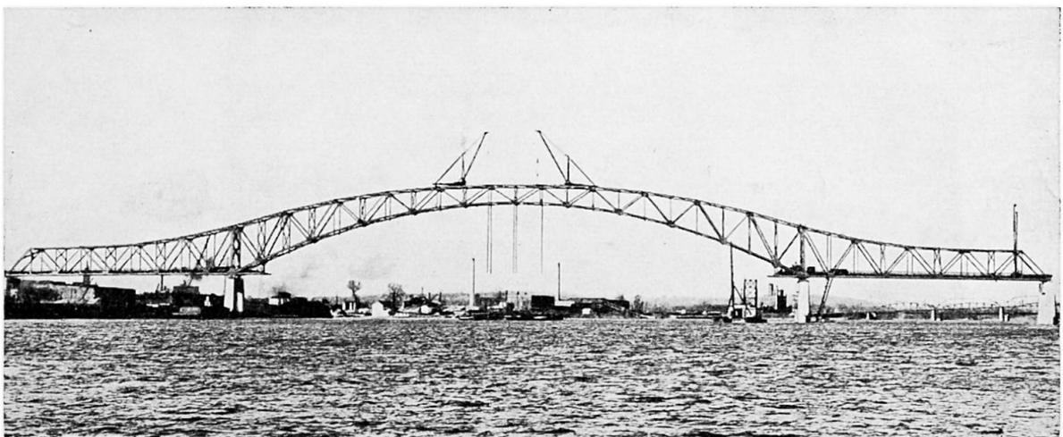
**Fig. 7.** Arch span fully connected.
