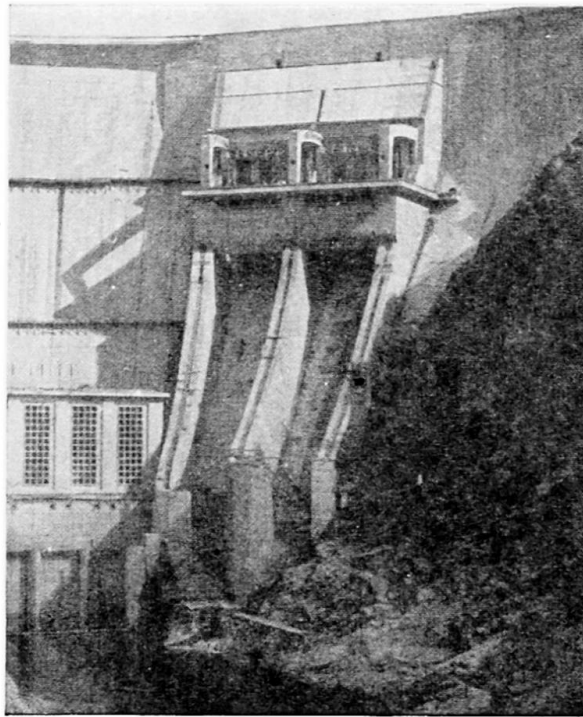
Fig. 13. Spillway of Castelo do Bode Dam
