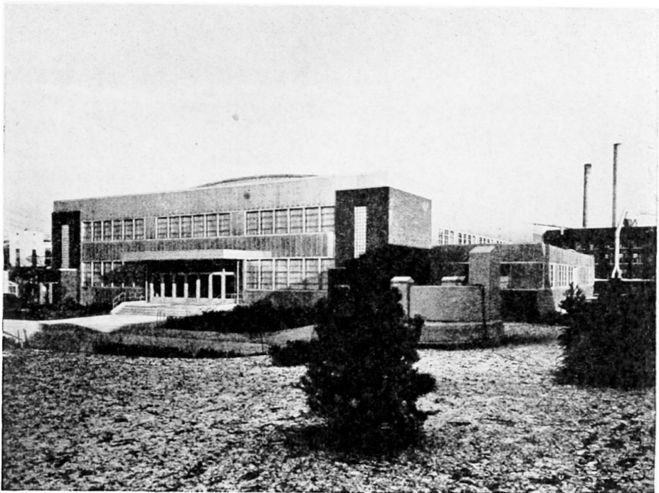
Fig. 15. Auditorium and recreation building. Light-gauge wall, floor and roof panels on conventional steel frame. Exterior sheet of wall panels is aluminium (Detroit Steel Products Co.)
