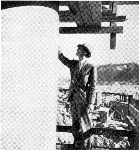
FIG. 12. Examination of the concrete surface of a column at Bergforsen
