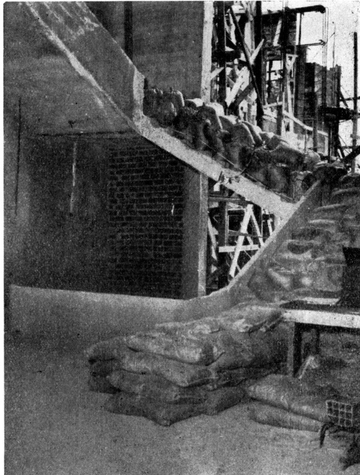
FIG. 8. Application of the uniform load
