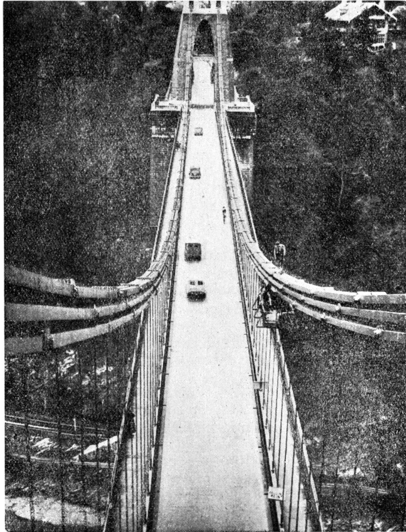
FIG. 1. View of suspension chains «Clifton Bridge». The cradle for metallising is clearly shown. Courtesy of Bristol Metal Spraying & Welding Co. Ltd.
