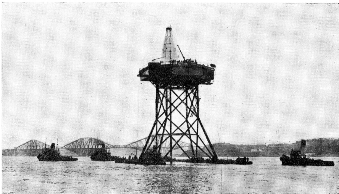
FIG. 9. Tower being towed out to its first drilling site
