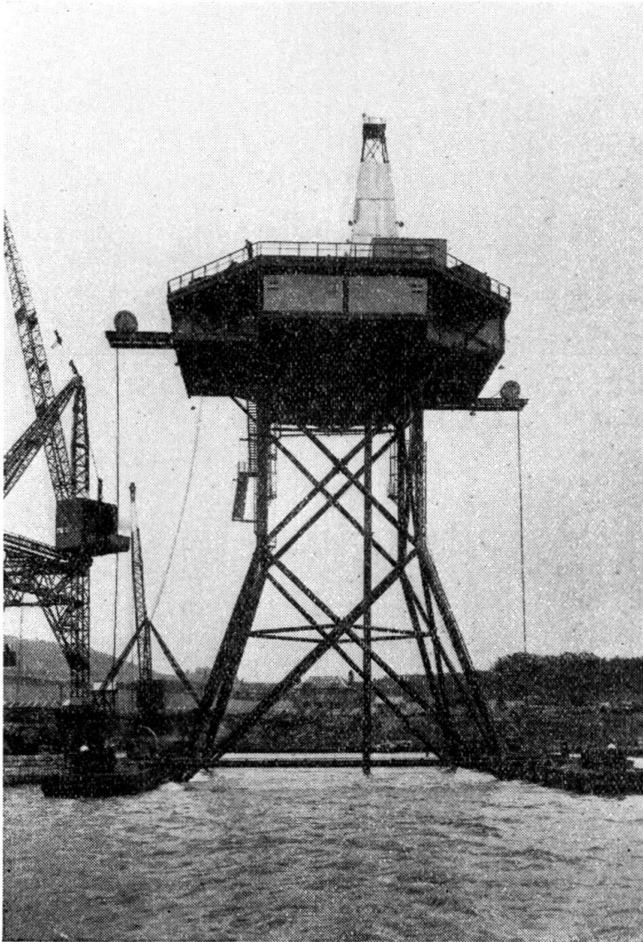
FIG. 8. Tower complete and ready for floating
