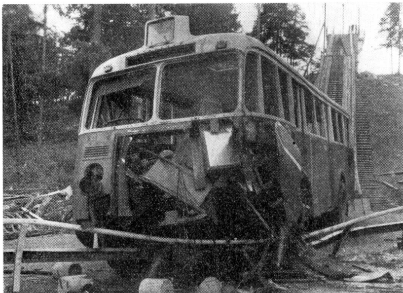
FIG. 11. Warding off parapet between roadway and cycle track after impact at an angle of 45°. Bus speed just before collision 48 km/h.
