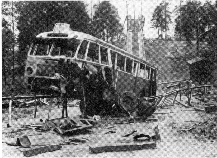
FIG. 10. The City's newly designed footpath parapet after impact at an angle of 45^\circ . Bus speed just before collision 48 km/h.
