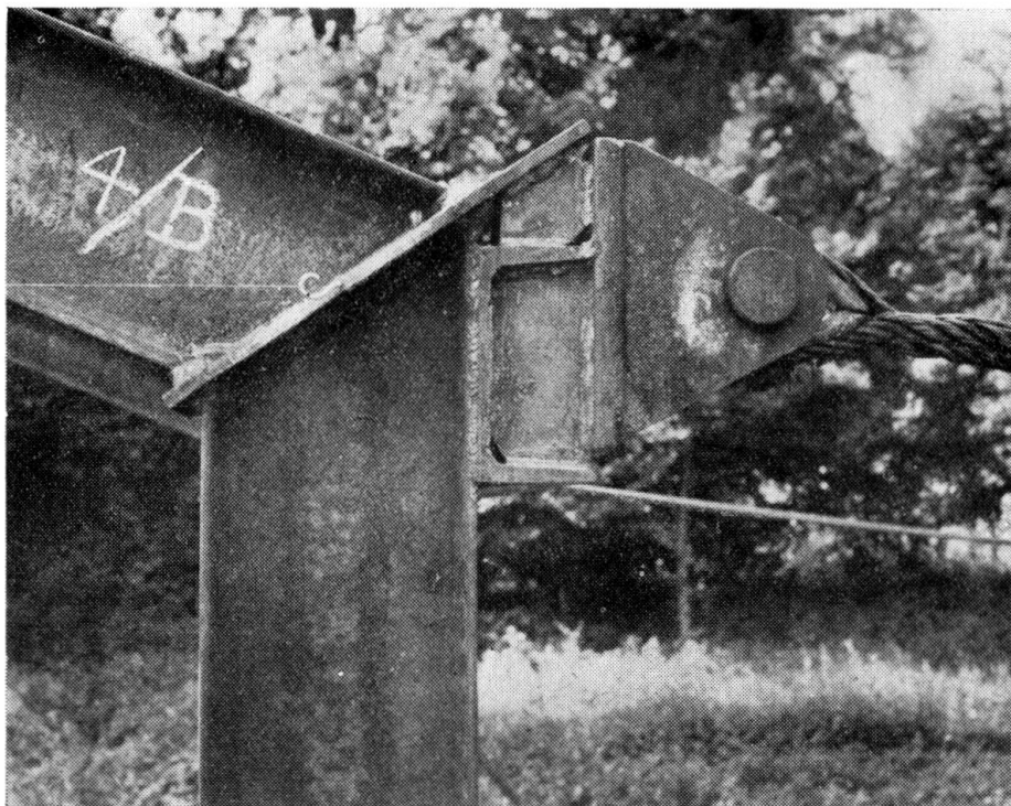
FIG. 3. Joint F, showing side load attachment
