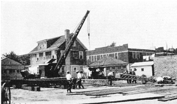
Fig. 4. Use of a crane is advisable to unload tools and equipment, and then to assemble and set up guy derrick.
