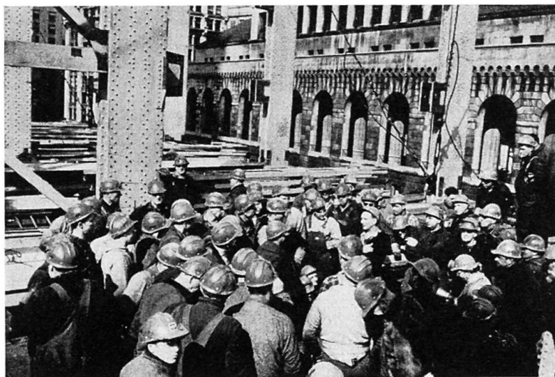
Fig. 17. Safety meetings should be held regularly, and safe operations result in efficient and economical production.
