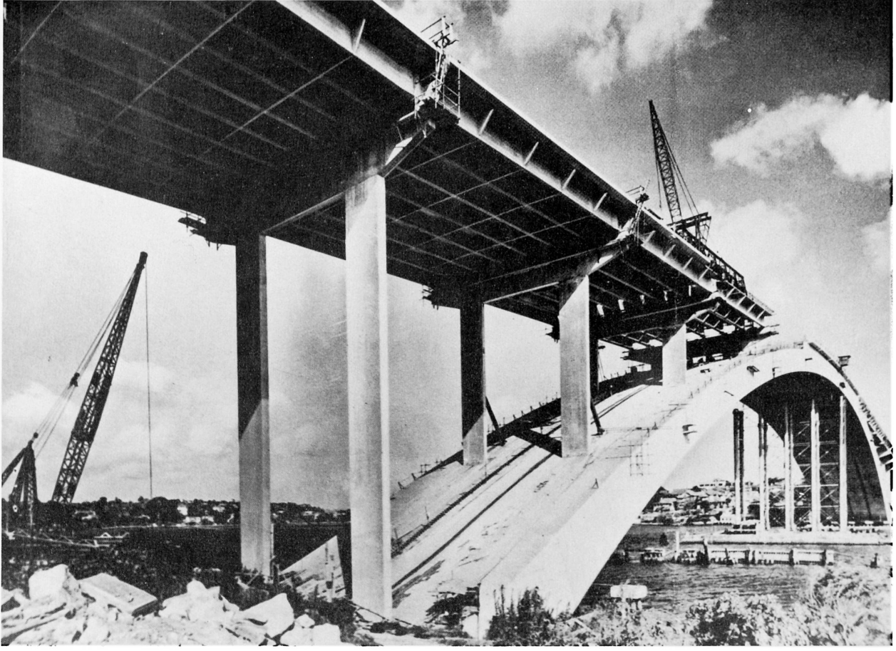
Fig. 7: Sydney Harbour and Distant Pacific — 2 ribs completed
