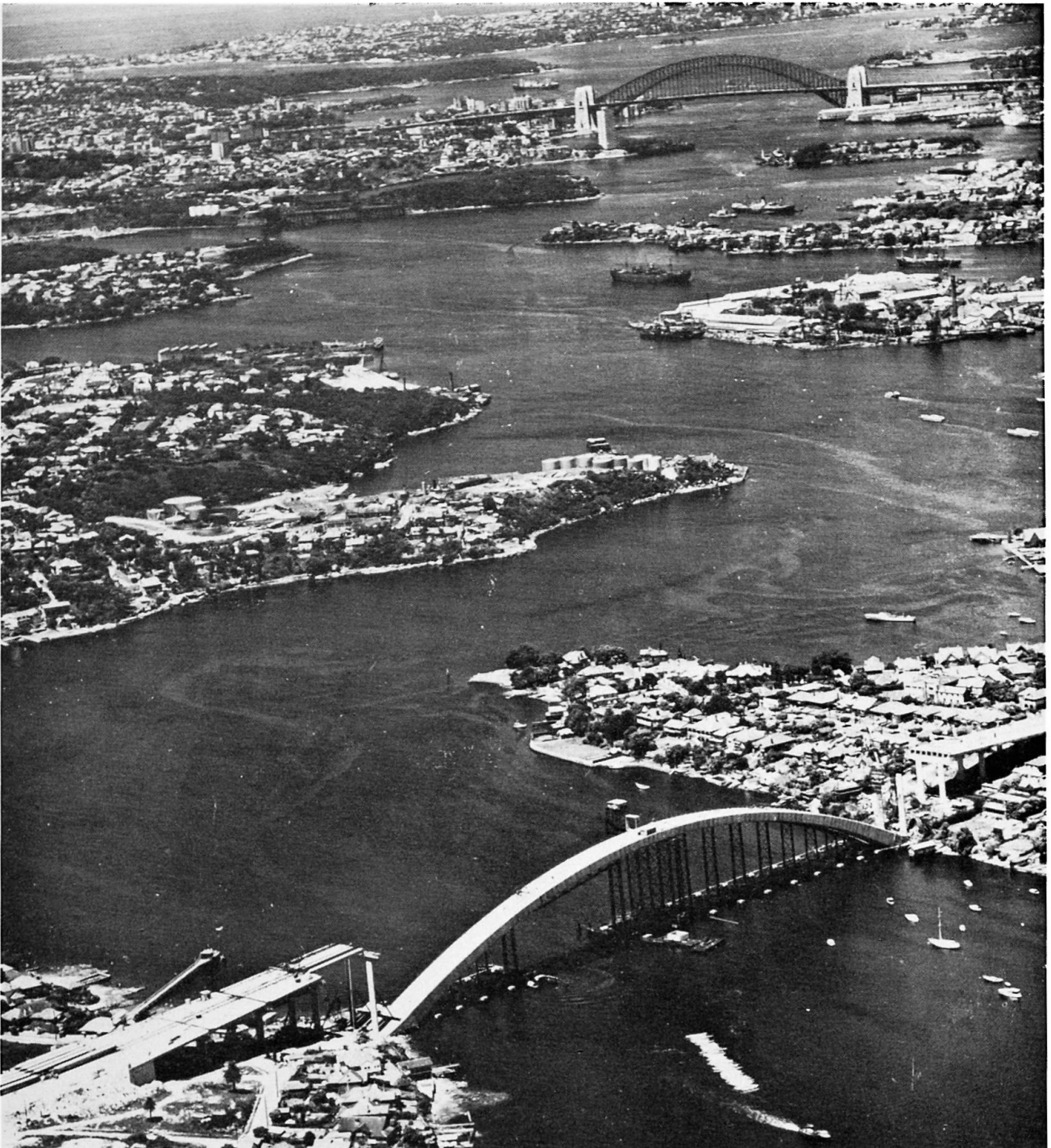
Fig. 8: Sydney Harbour and Distant Pacific – 2 ribs completed
