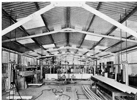
Fig 11. Plastic collapse of sheeted building.
