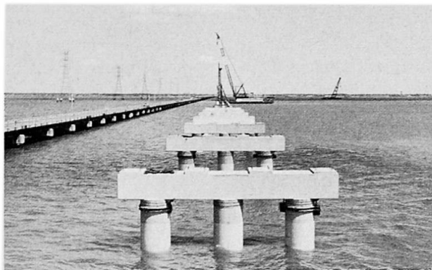
5. Newly installed piles and caps for replacement roadway
