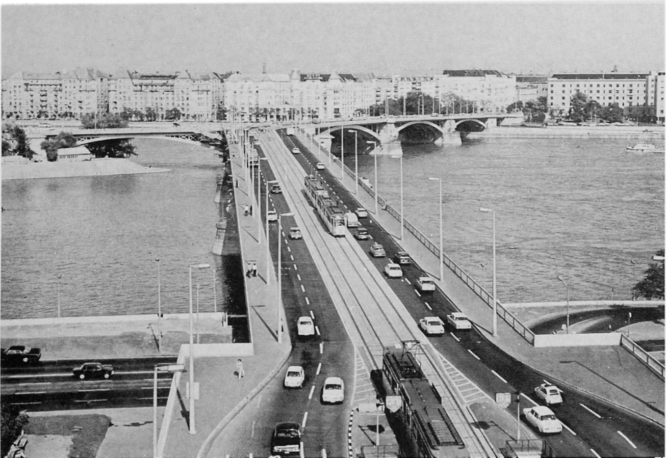
Fig.2. The Margit bridge after renewal.
