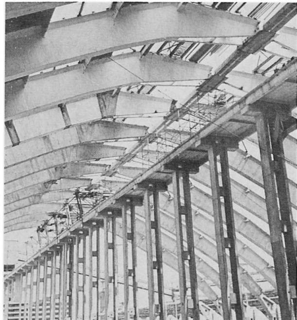
Fig.10 Inside view of the depot
