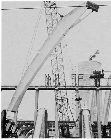
Fig.5. The handling of the precast element
