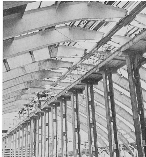
Fig.10 Inside view of the depot
