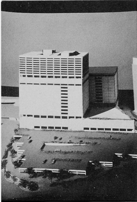
APPAREL MART AND HOTEL: This composite steel and concrete structure comprises a hotel and an apparel mart with 125,000 square meters of space.
