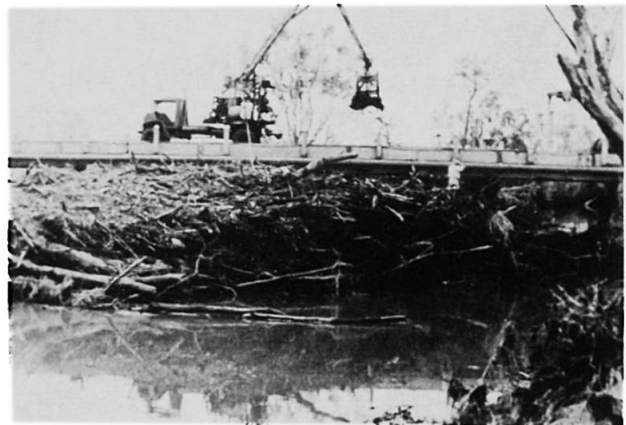
Figure 2 Spans too small Deck at flood peak
