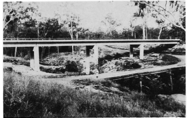
Figure 4 Submersible bridge replacing lower timber bridge
