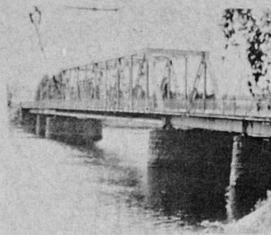
The existing steel truss bridge with a span of 131 m and a width of 10.5 m. Completed 1933.
