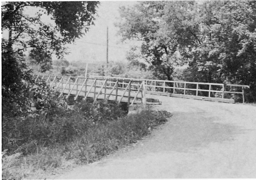
Photograph 1: Case Study 1 - Bridge prior to renovation.
